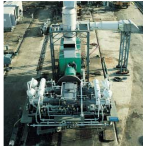
GE PGT5 gas turbine driven compressor during full load test.
