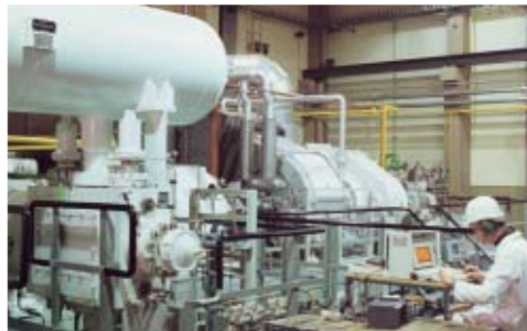
Compressor field monitoring.
