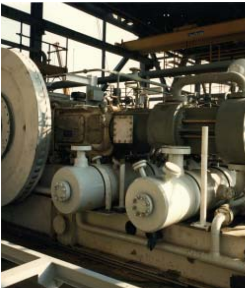
Re-injection compressor - model 6HE/2 at 415 bar.
