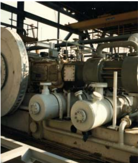
Re-injection compressor - model 6HE/2 at 415 bar.
